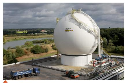
Formed segments welded together to make a complete sphere. Fitting and quality is an absolute requirement. Sphere in the picture is nearly 26 meters in diameter
